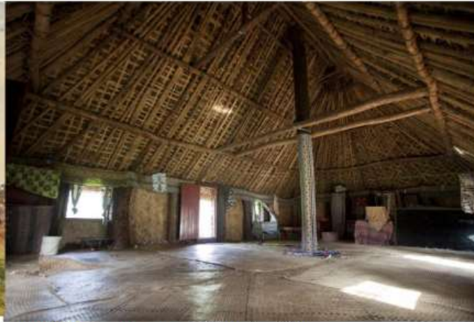
Typical Bure Structure - Interior View
