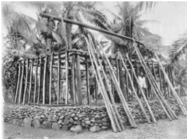
Figure 8 Yavu (Foundation of a Bure)
