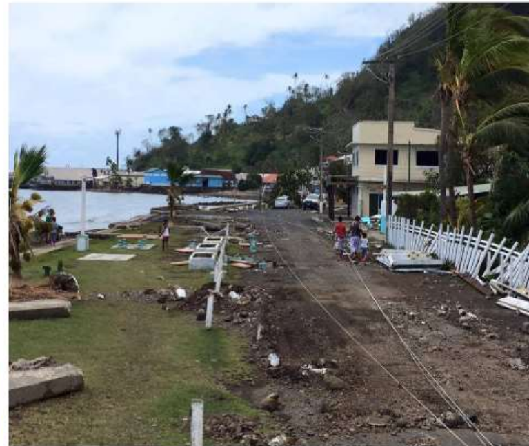
Beach Street view towards Pafco- Cyclone damages
