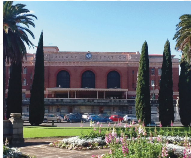
Figure 2: Façade of Gummer and Ford's Auckland Railway Station. Photograph: Cameron Moore
