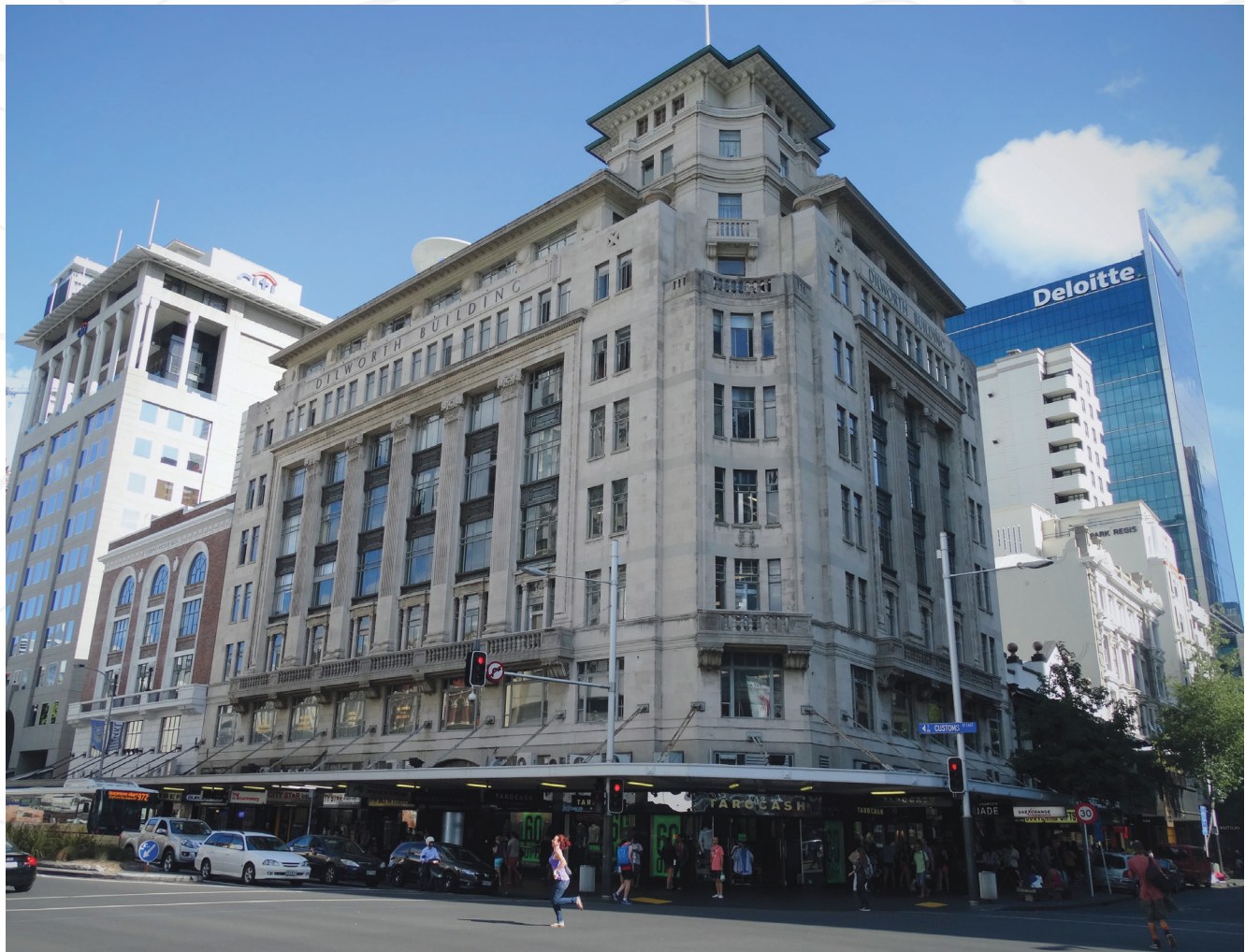
Figure 4: Gummer and Ford, Dilworth Building, 1825–27, Auckland. Photograph: Cameron Moore
