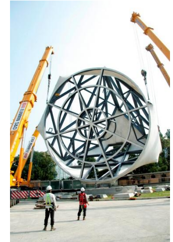
Figure 2- The Prada Transformer
