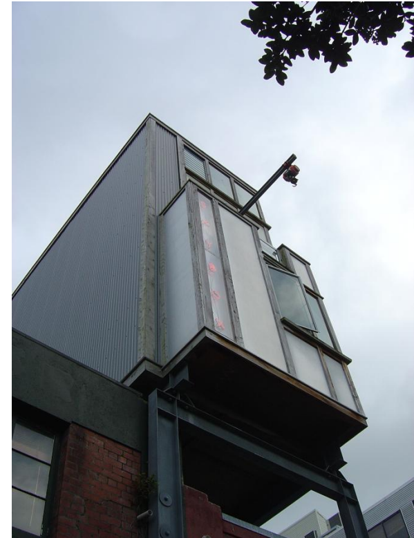
Figure 45 – Exterior view of Skybox straddling the building below
