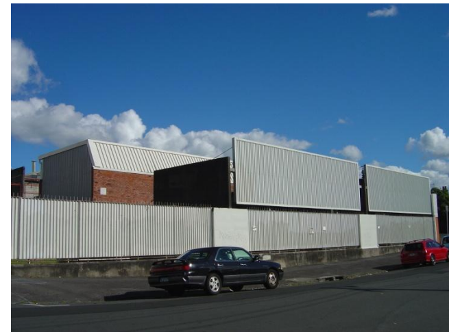
Figure 11 – View of site from Kingsland Terrace
