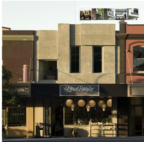
Figure 3 – RTA building illustrating borrowed proportions from neighbouring buildings
