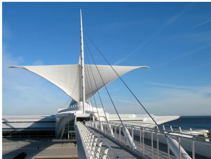
Figure 14. Santiago Calatrava’s Quadracci Pavilion which features roof fins that open.
