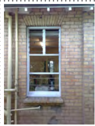
Building 06 - Windows and services
