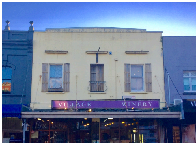
Figure 1: Mt Eden URM Building
