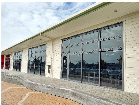
Figure 2. Retrofit school building.
