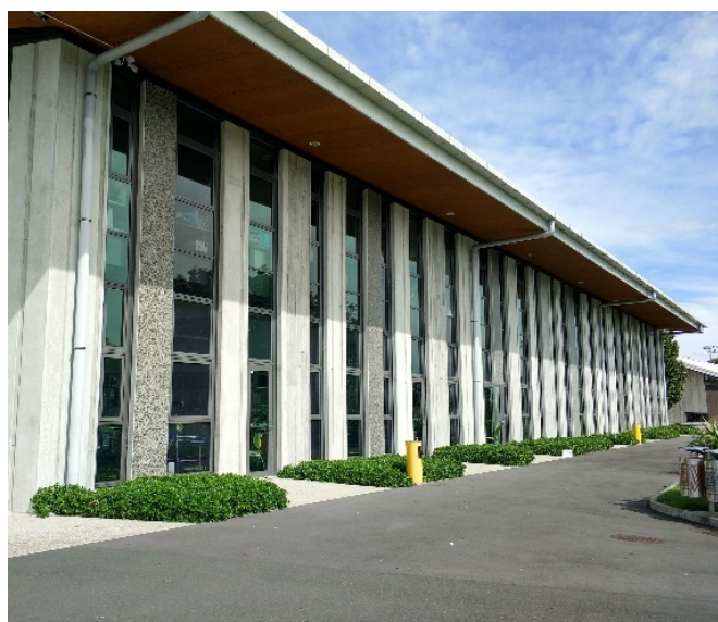
Figure 3. New school building with precast insulated concrete panel wall.
