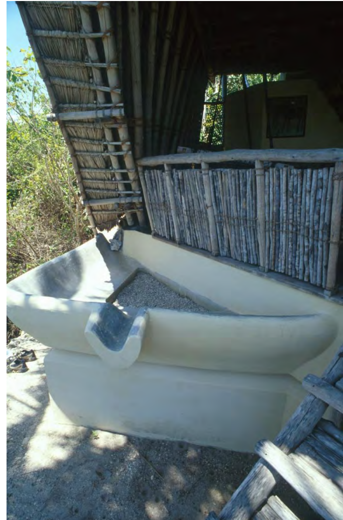
Figure 33: Rainwater Collection and Filter
