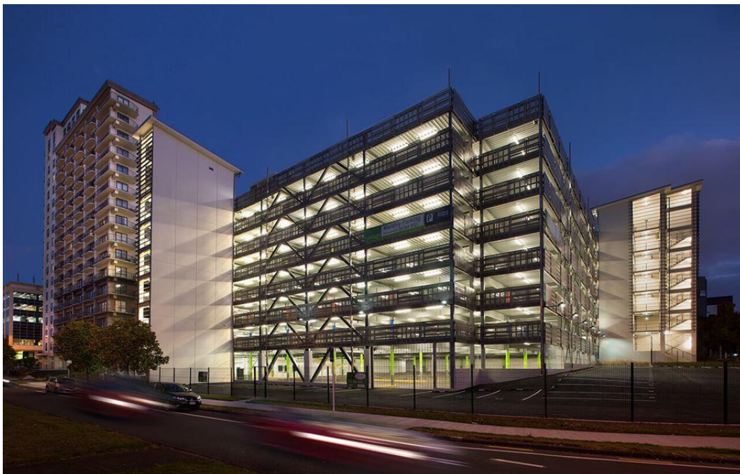
Figure 46: Ronwood carpark building
