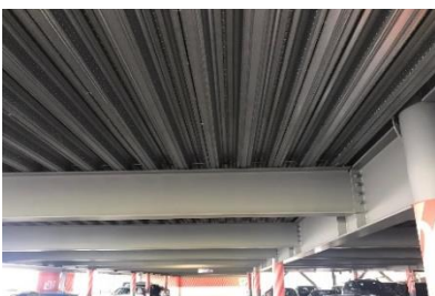
Figure 52: Comflor and steel structure
