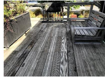
Figure 24: Decking materials are made out of salvaged waste materials
