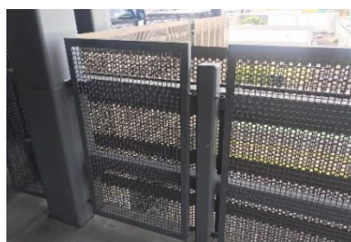
Figure 51: Steel mesh balustrade
