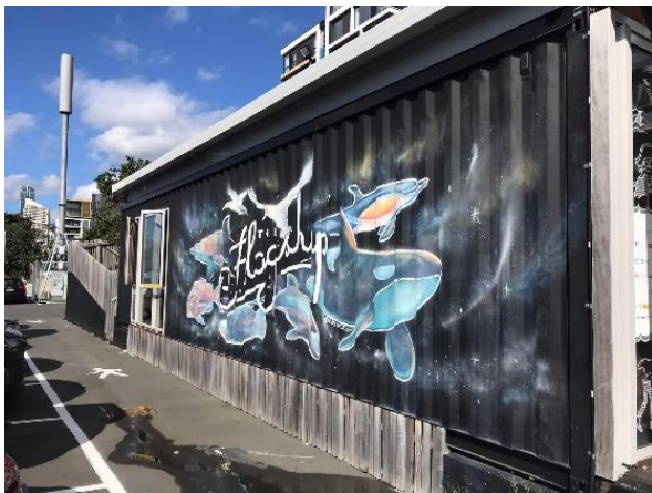
Figure 22: Shipping containers donated and utilised as building elements
