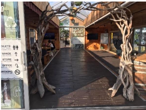
Figure 27: Interior linings and flooring made of salvaged timbers
