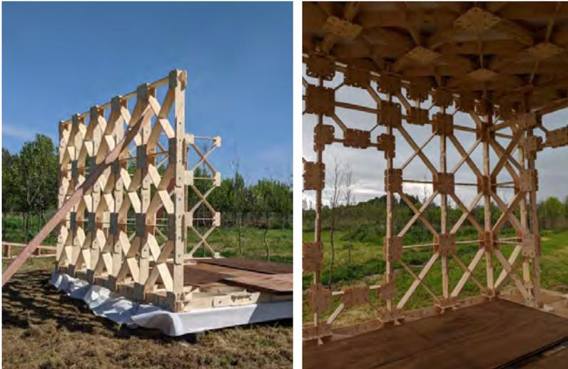
Figure 2. Wall Frame and Sub-Floor during Assembly
