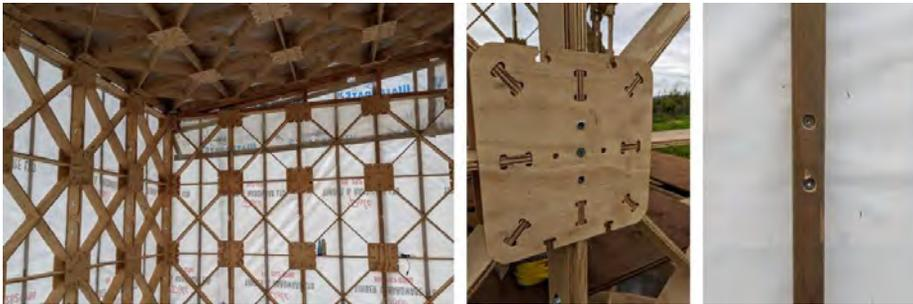
Figure 3. Synthetic Building Wrap (non-woven thermally bonded polypropylene) over the modular frame (left), the cavity batten mounting points (middle) and the batten installed (right).
