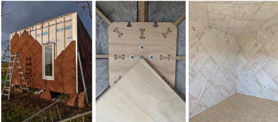
Figure 4. Installation of the Thermally Modified Plywood Cladding (left), a close up image of the pressure clip receptacle used for the internal linings (centre) and the finished lined interior (right).
