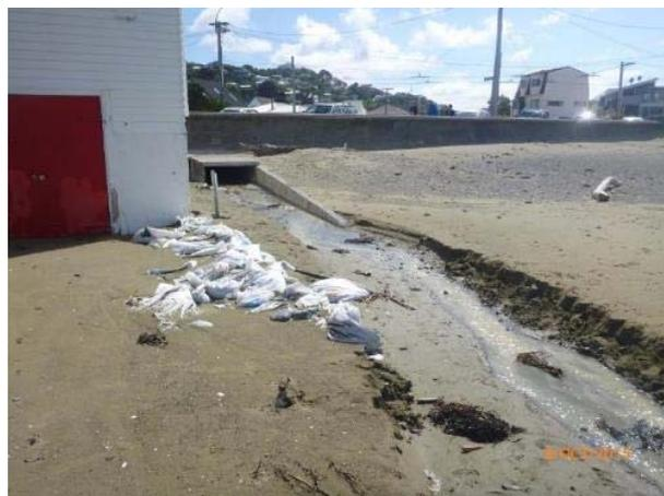
Figure 10 The stormwater outlet next to the Maranui SLSC is one of the most troublesome in Lyall Bay; it outfalls at the base of the seawall (i.e. is the more landward than others), is very close to the building and has a relatively high discharge rate compared to others. Burying and lengthening to the intertidal zone will reduce the negative impacts on beach stability and amenity.
