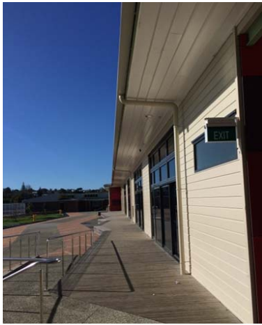
Fig. 3 One-story building with light rain screen wall
