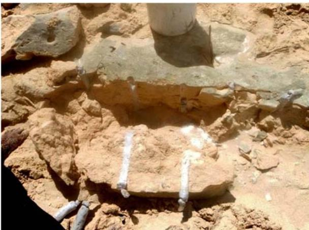
Figure 11. A 350 mm deep section of limestone cracked off the construction 'face' with Expando.
