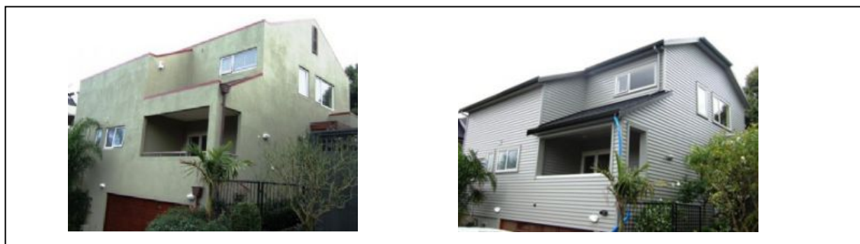
Figure 2: Reliant Group. Before and After Re-cladding Examples [9]
